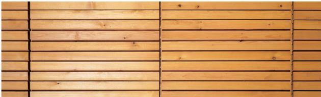
Available with overlapped or profiled sections. The board profile and spacing can provide a variety of design effects, as well as protection for the building. If using horizontal boarding, consider how the boards will be fixed and jointed to provide good detailing for the building. Tongued and grooved boards should be installed tongue upwards.
